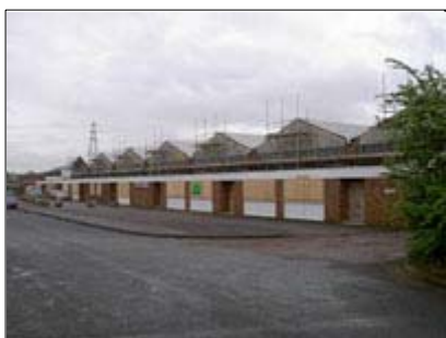
The property pre-refurbishment – July 2005
