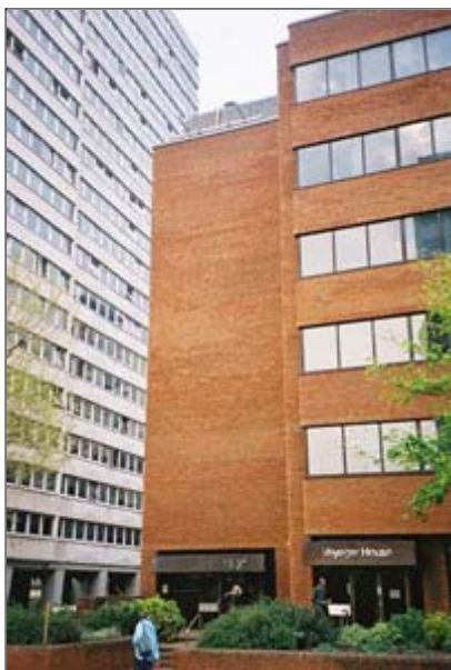
Voyager House, Croydon prior to refurbishment in June 2004
