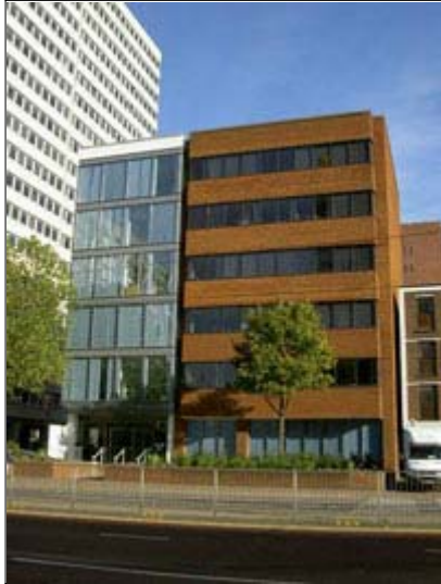
Voyager House, Croydon following refurbishment – November 2005
